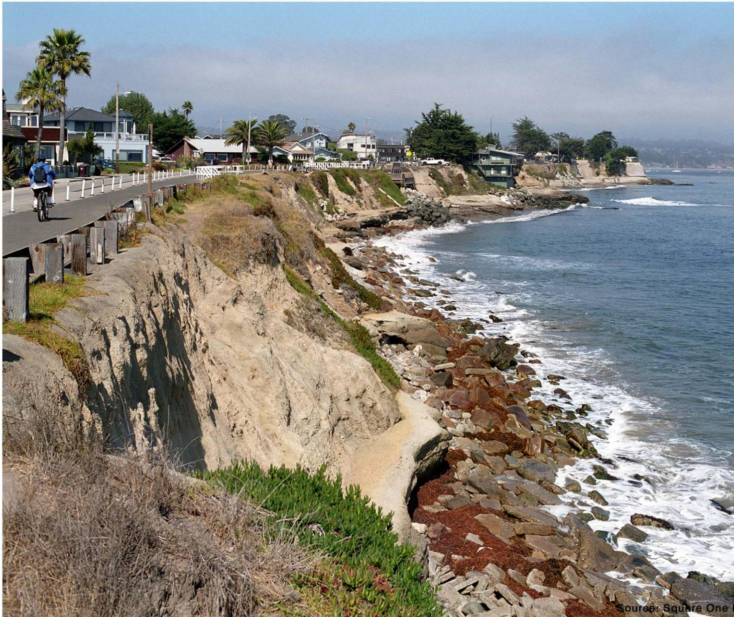
Existing conditions at the project area include concrete rubble, sculpted and colored soil nail walls constructed as emergency repairs in 2004 (lower left-hand corner of picture), white protective railing around areas of failed roadway, nonnative vegetation and minimal beach area due to the concrete rubble and rock riprap.
